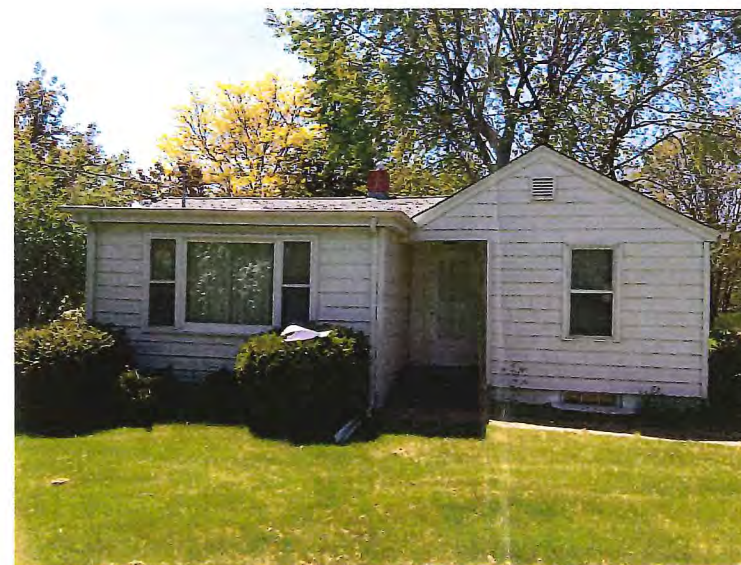
VIEW OF FRONT (EAST SIDE) OF HOUSE
