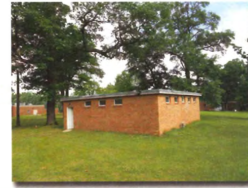
EXISTING RESTROOM BUILDING
