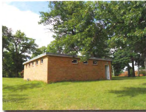
EXISTING RESTROOM BUILDING
