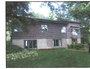
WEST (LAKE) SIDE OF 5107 ALAMEDA STREET
