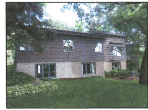
WEST (LAKE) SIDE OF 5107 ALAMEDA STREET
