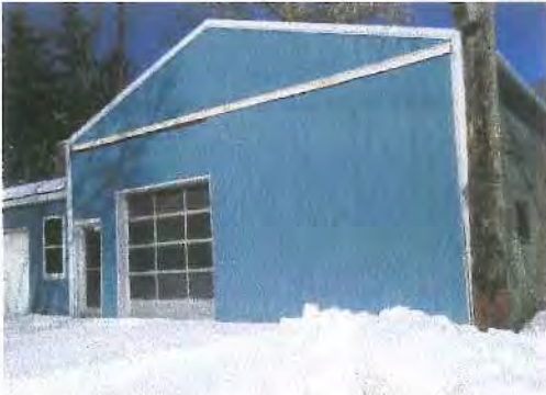
Close up Existing Detached Garage (to be removed)
