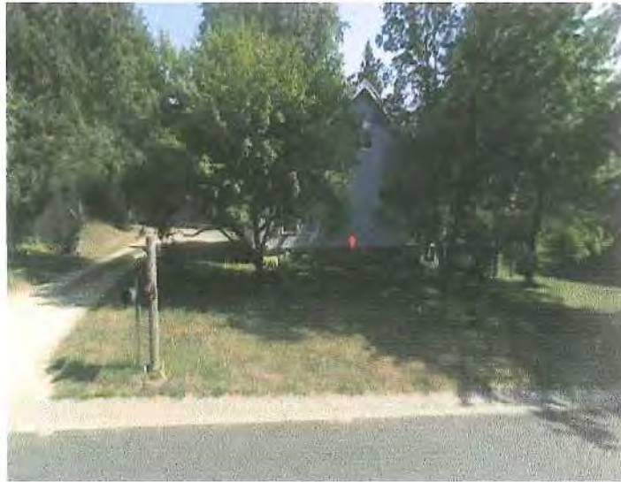
View of house from street. Note house does not face street.
