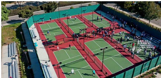
Pickleball with fence-mounted noise mitigation (photo of Poinsettia Community park by acoustiblok.com)
