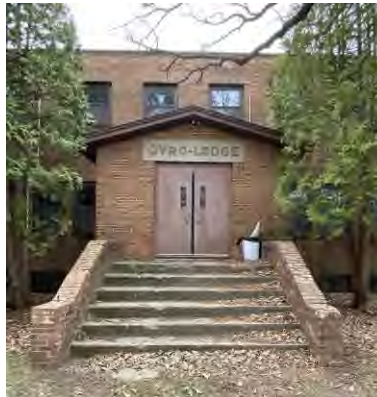
Fig. 5. Gyro Lodge main entrance, east elevation. (May 2022)
