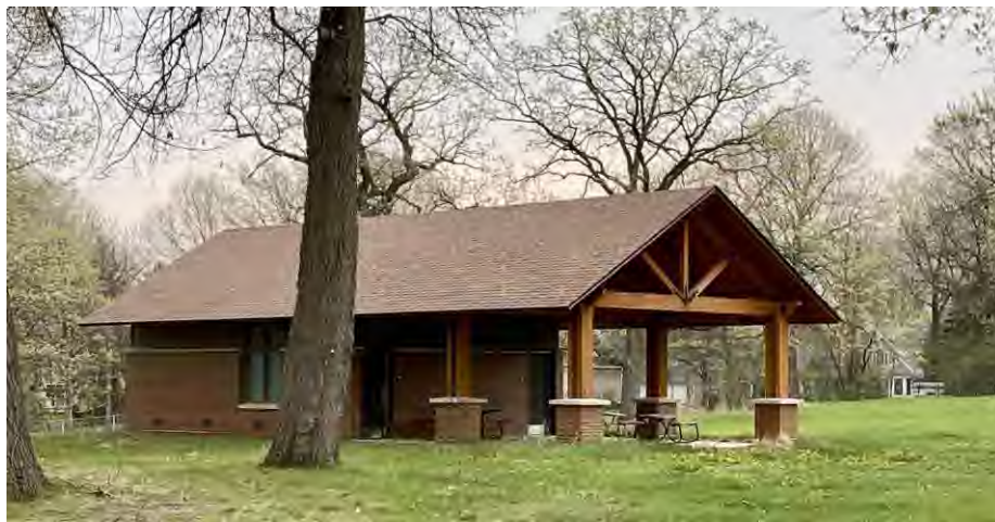
Fig. 8. Restrooms, north and west elevations, facing southeast. (May 2022)
