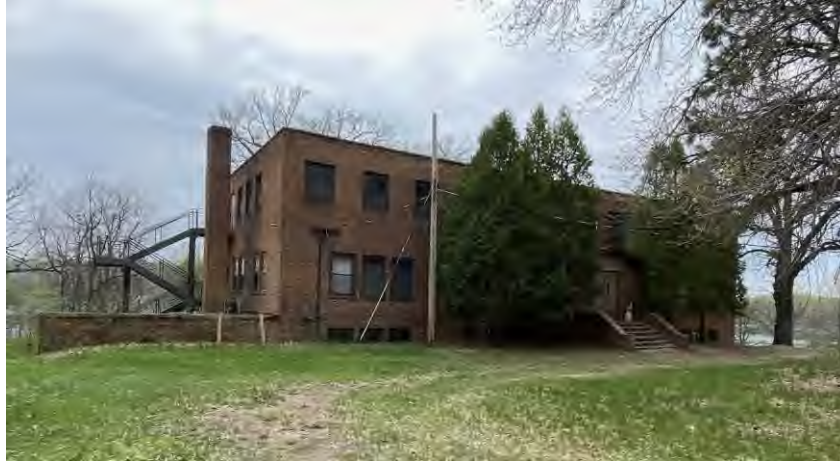
Fig. 4. Gyro Lodge, east elevation, facing west. (May 2022)
